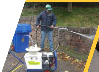
WET SAND BLASTING
